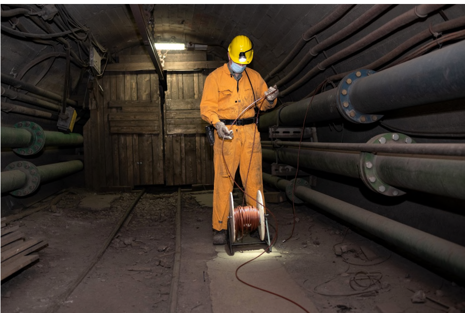
Cable installation in the Velenje Coal Mine.
